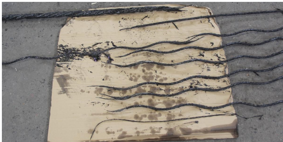
Fig. 4. Degradation of the metal core of the lifting rope of the SchRs excavator lifting system as a result of the torque (photo A. Tytko)
